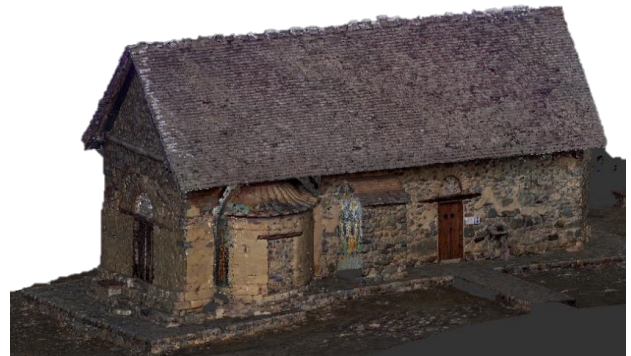
Figure 2: 3D Model of Asinou Church with texture mapping using the produced photogrammetric images. Images were processed with Agisoft Photoscan.
