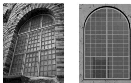
Figure 4: (left) Picture of a modern reconstruction of a window in the Constantinian Baths at Arles (credit: J.W. Humphrey). (right) The reconstructed north window of 4W showing the adjustable space between panels.
