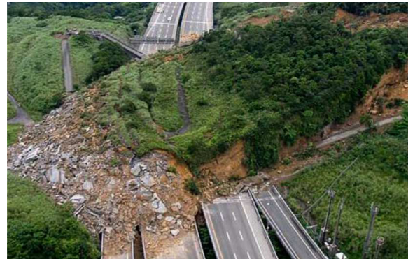
Figure 1: Example of mass movement erosion in real world.
