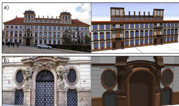
Figure 1: Front facade of (a) the Tuscany and (b) the Thun-Hohenstein Palace in Prague. On the right side are facades created by CGA shape grammar.
