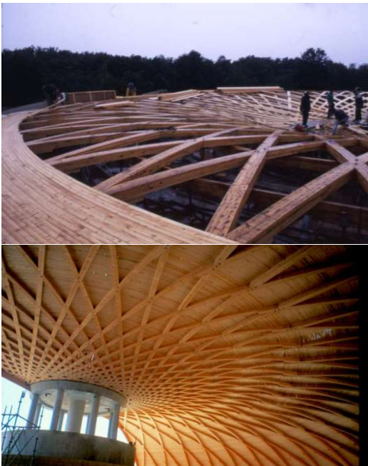
Figure 17: realization, outside and inside
