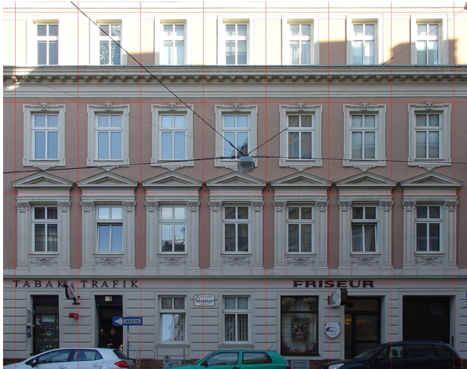
Figure 4.1.: The red lines indicate the grid, which has been detected on the façade. The proposed algorithm is robust to obstacles such as different illumination or reflections in the windows (best seen in color).
