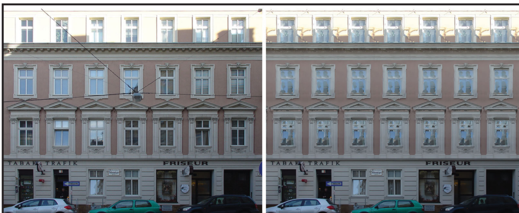
Figure 6.9.: A failure case of our algorithm. In the upper story the outlier rejection method could not determine the actual wall color coherently, which results in destroyed structure of the original image..
