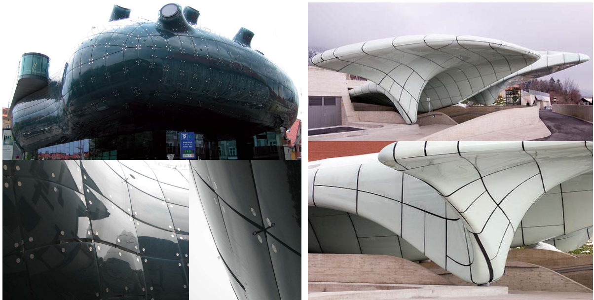
Figure 4.2 Projects involving double-curved panels where a separate mold has been built for each panel. These examples illustrate the importance of the curve network and the challenges in producing architectural freeform structures. (Left: Peter Cook and Colin Fournier, Kunsthaus, Graz. Right: Zaha Hadid Architects, Hungerburgbahn, Innsbruck.)
