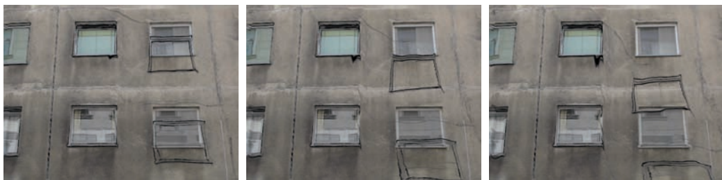
Figure 2.8: Caricaturistic visualization of a facade deformation. The image of the deformed facade is overlaid by the caricatures. The exaggeration parameter is increased from left to right.
