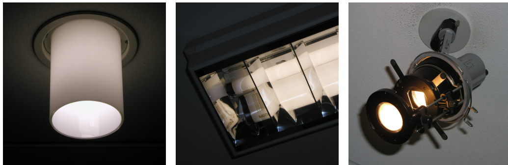
Figure 2.4: Common elements to modify the radiation pattern of a luminaire. Left: A lamp screen with diffuse transmission. Middle: Office lamp with reflective components. Right: Spotlight with polygonal aperture and projective lens.
