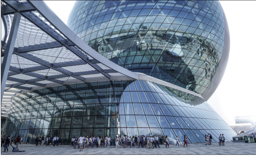
Figure 2.6: Side detail of Nur Alem , the main pavilion of the Astana EXPO 2017 Exhibition in Astana, Kazakhstan. Mostly cylindrical panels were used to rationalize the curved transparent freeform façade (different from the sphere).
