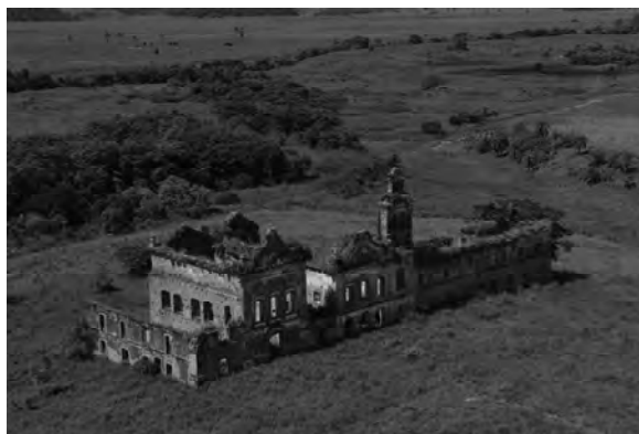
Figure 1: Ruins of São Boaventura Convent, before the propping process.
