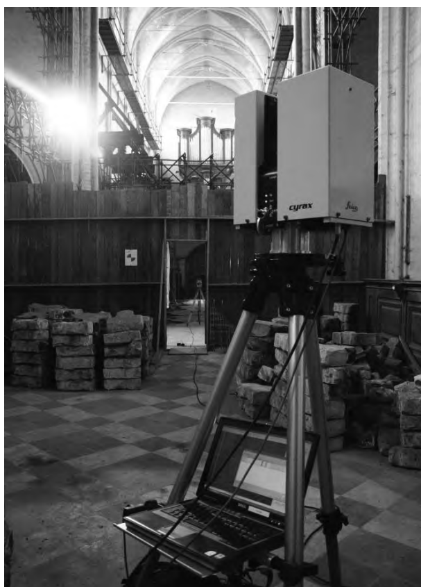
Figure 1: Scanning of the masonry vaults, St.James Church (Leuven, Belgium), author.
