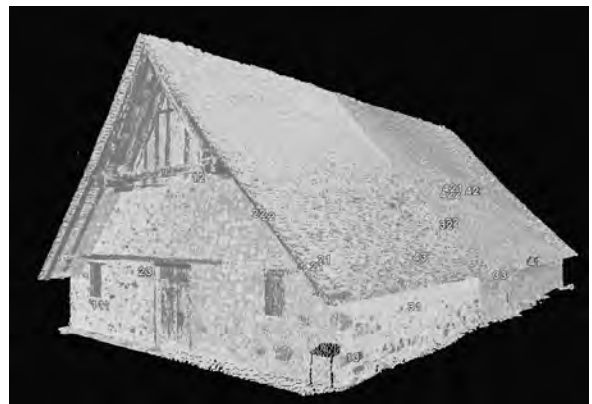
Figure 9: The complete point cloud of the Church of Podithou
