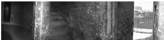
Figure 3: A view from the inside of the signal light tower, showing the spiral staircase and the balcony on level 3 (UMR MAP, 2006).
