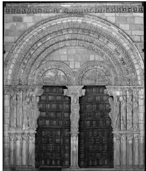
Figure 11: Printing quality final orthoimage, seamlessly composed from five different layers after radiometric equalization
