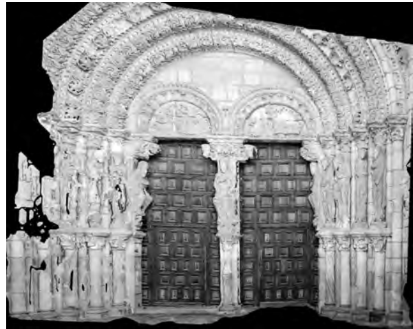
Figure 9: Synthetic image SBA from disparity map. Overlaps almost exactly with image A, but image information comes from image B
