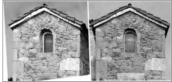
Figure 1: Simple façade. Two plane rectified images. Differences are evident at the window but smaller errors are also present everywhere.
