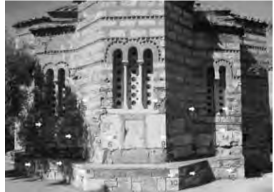
Figure 7: Target positions measured on the façade
