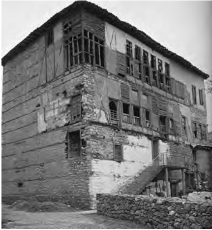
Figure 1: Typical earth –block masonry of the 19 th cent. in Veroia, Greece (Papayianni, 2006).
